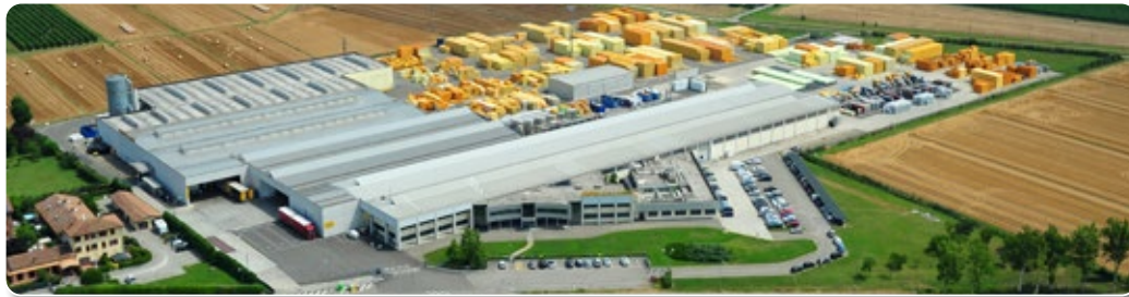
HEADQUARTERS DUNA-CORRADINI Spa (Soliera - Italy)
